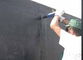
**10** - Fasten the bituminous membrane to the wall using the appropriate mechanical fastening systems at the overlapping points.
