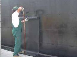
**5/6** - AApply the membrane sheet by first fastening the upper part on the wall and then proceeding downwards.
