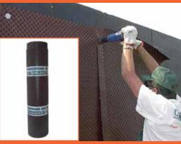
**11/12** - Apply mechanical protection (e.g. POLYFOND KIT or POLYFOND KIT DRAIN, HDPE dimpled membranes) over the waterproofing membrane if necessary.
