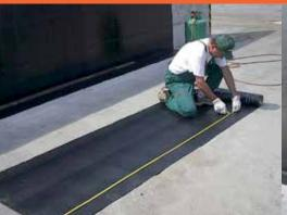
**4** - Cut the membrane sheet to the size of the surface to be waterproofed.
