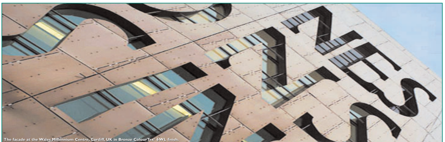
The facade at the Wales Millennium Centre, Cardiff, UK in Bronze ColourTex® 6WL finish.
