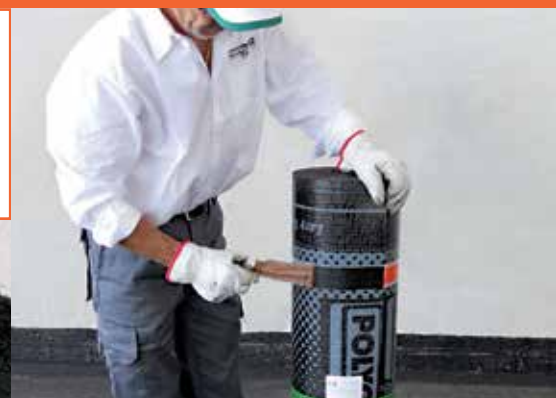
3 - Completely strip away the product identification tape.
