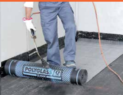
5 - Position and apply the sheet by flaming its bottom surface.
