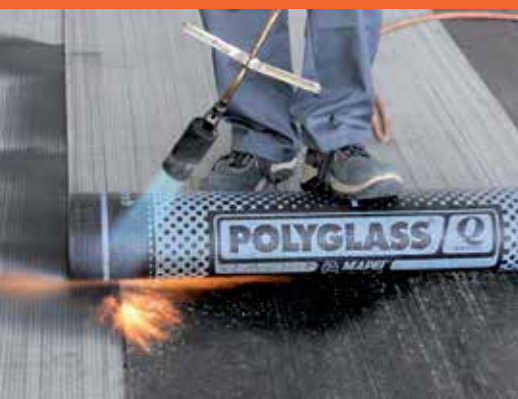
7 - Apply the second sheet with adequate overlapping.
