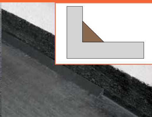
2 - Position the corner border near the horizontal-vertical joint.
