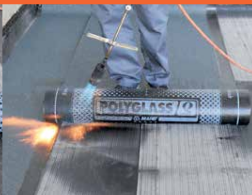
8 - Lay the second layer by overlapping. Do not cross the sheets.
