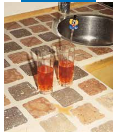
An example of a bonded and grouted kitchen worktop
