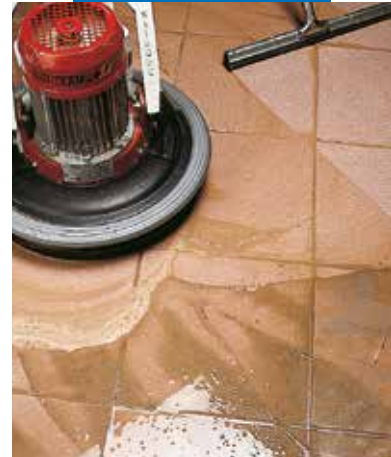
Finishing a porcelain tiled floor with single-brushed power float or rubber squeegee
