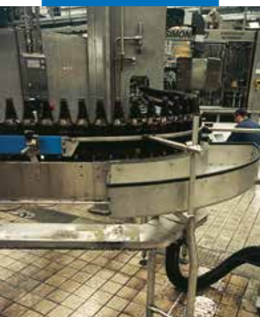
An example of a grouted brewery floor
