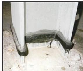
*Unlike PVC waterstops, WATERSTOP-RX can easily be installed around irregular structural elements.*
