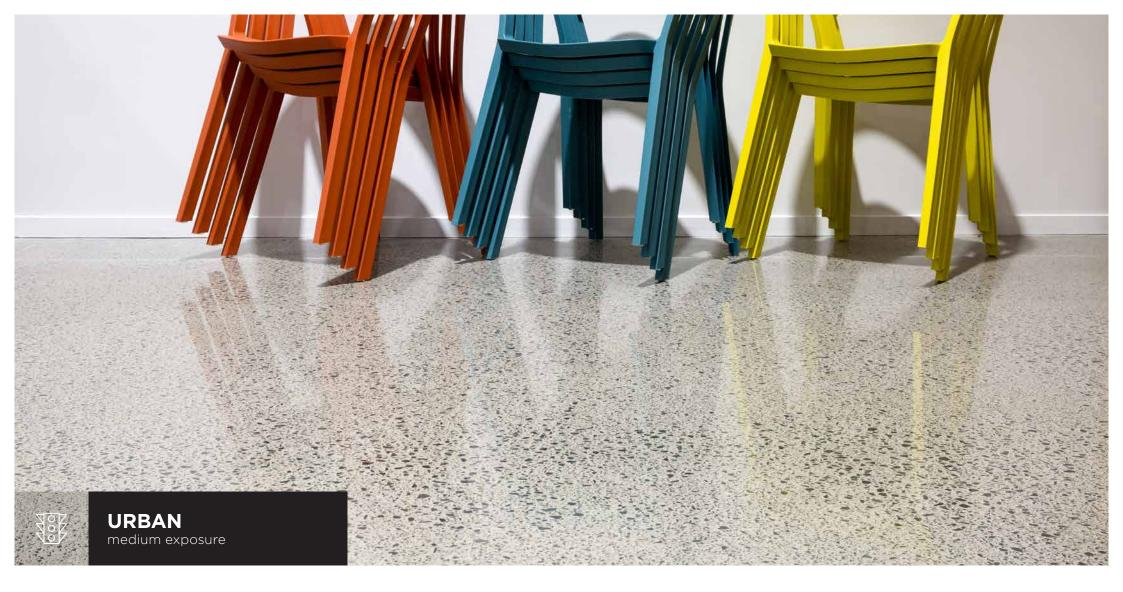
URBAN is the most traditional diamond polished finish combining cost effectiveness with an excellent random stone exposure. It requires the removal of the 2-3mm of the concrete laitance to reveal the underlying aggregates. The floor iis ground flat leaving a random mix of medium stone and fine aggregates that are then polished with resin diamonds.
