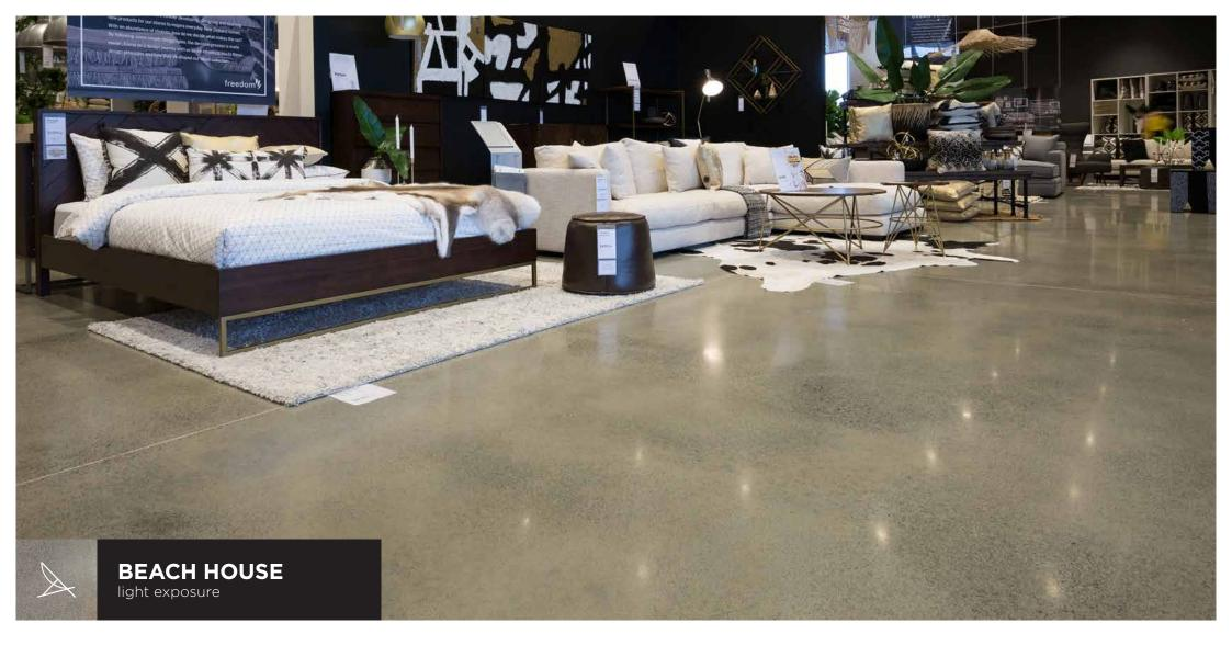
BEACH HOUSE is a classic salt & pepper diamond polished finish. It requires the removal of 1-2mm of concrete laitance to reveal the underlying fines. A lightly ground floor incorporates the natural contours of the concrete, with the addition of a resin diamond polish. Ideal for newly laid floors where placing can be controlled to achieve a flat surface.
