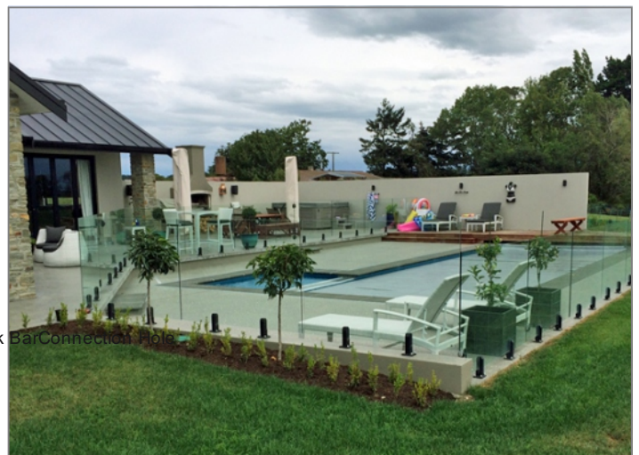
Juralco Edgetec Mini Post Framless Balustrade Top Fix to Tiled Concrete Deck. Pool
