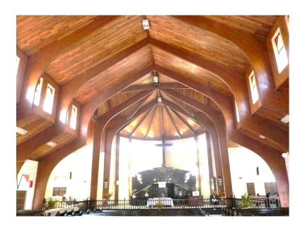
**Site Assembly** - Members arrive on site in the form of half portals; wpith the use of a mobile scaffold to support the apex. Erection is quickly achieved by lifting the half portals into position onto holding down bolts and aligning the simple bolted apex joint. An average of 6 to 10 portals can be fully erected in a working day. Each frame can be temporarily braced longitudinally so that a secure structure is available for cladding and roofing.
