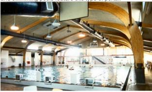
**Solid Knee** - The gap left between the curved knee section in the open knee portal and the upper wall and roof line is eliminated in this style. The shape of this portal follows the wall and roof profile on the top side, while giving a sweeping curve on the inside.
