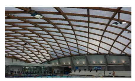
Cranked Beams - These beams follow the roof pitch on their top edge while the bottom forms a radius curve. Cranked beams taper from the tangent point to a minimum end depth to provide maximum economy. They may be simply supported on timber or concrete posts.
