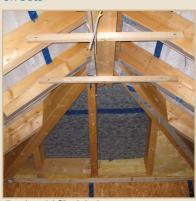
Different products installed: Microporous membrane - Nonporous SOLITEX TEEE
