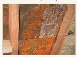
Without moisture management there is a risk of water condensing in the building envelope, and thus a risk of structural damage and mould.
