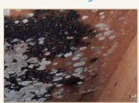
Constructions that are not airtight do not only result in mould on the inner surfaces of structural components, but also in mould within the construction.
