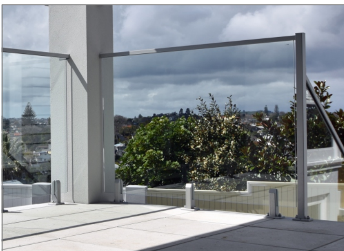
Juralco Edgetec Mini Post showing the Interlinking Top Rail and the use of a Top Mounted Edge Post and Brackets back to the structure
