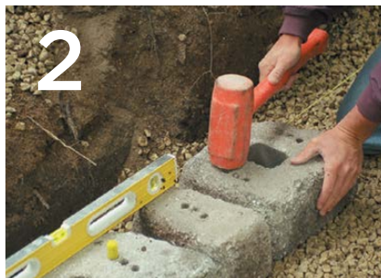
2 INSTALL THE FIRST COURSE & PINS
