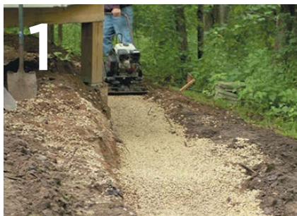
1 PREPARE THE BASE LEVELLING PAD
