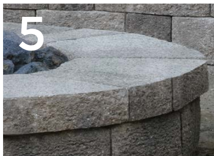
5 CAP THE WALL
