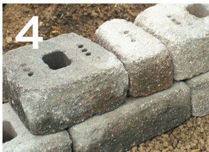
4 INSTALL ADDITIONAL COURSES (NO MORTAR REQUIRED)
