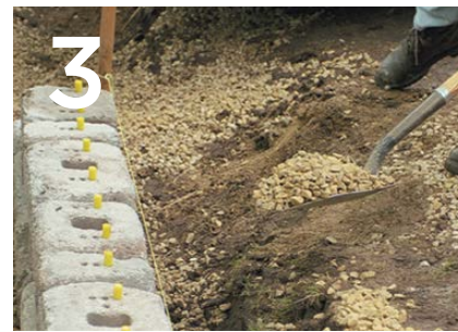
3 BACKFILL & COMPACT
