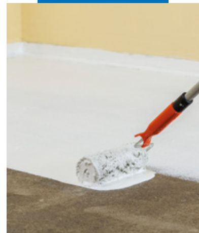
Application of the first coat of Aquaflex Roof Premium on cementitious screed
