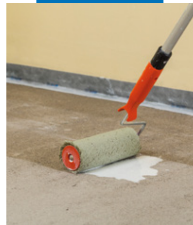
Cementitious substrate primed with Mapecoat I 600 W
