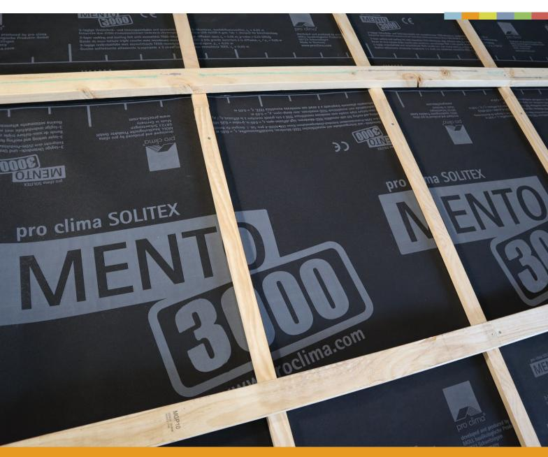
Weather Resistive Barrier for Weathertight Roof Systems
