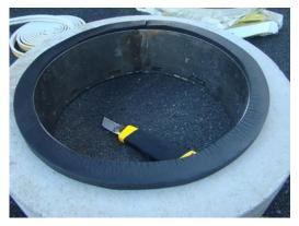
Photo 2: Soft closed cell foam on base of concrete ring.
