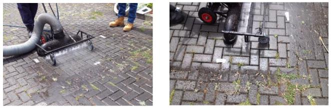
Photos 4 (left) and 5 (right): Cleaning the pervious surface. The thirteen, 1,000 psi water jets dislodge the sediments/moss/weeds from the surface and in the joints, which are then picked up with the vacuum suction. Most weeds are dislodged and vacuumed up but some weeds with long roots remain and need to be hand plucked.
