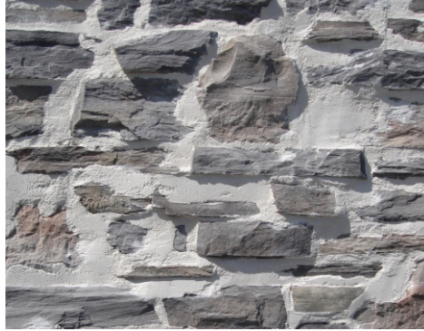
WC Alex with White Overgrout
