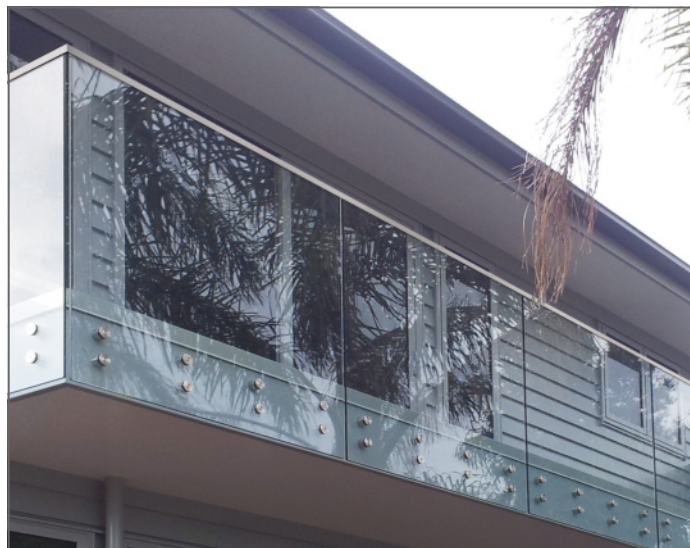
Edgetec Double Disc SS, C/S screw fixings with Top Interlinking Rail
