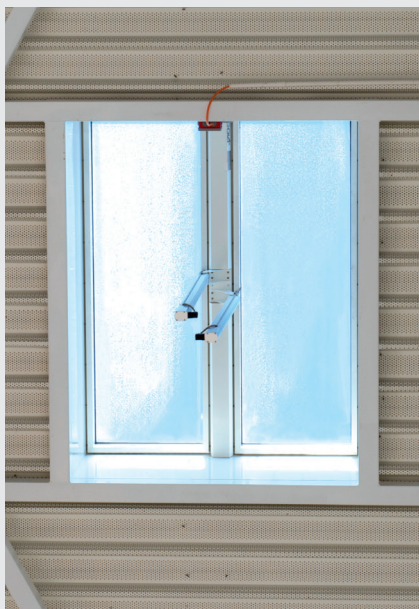
Firelight brings daylight into the building through its glass or polycarbonate lids.
