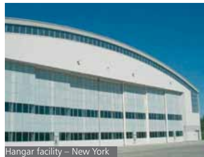
Hangar facility – New York
