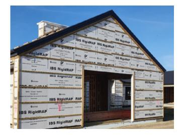
IBS RigidRAP<sup>®</sup> comprises of an 8mm thick, moistureresistant, oriented strand board (OSB3) panel with a synthetic wall underlay adhered to the outer face, suitable for use as a wall bracing element, structural rigid air barrier.
