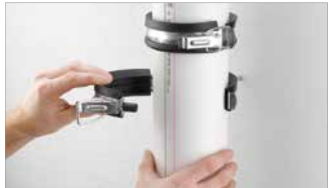
Fig. 7-16 Closing supporting bracket.
