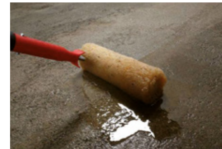
Application of waterproofing primer on a damp substrate
