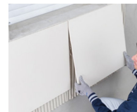
Installing ceramic on a vertical surface with thixotropic adhesive
