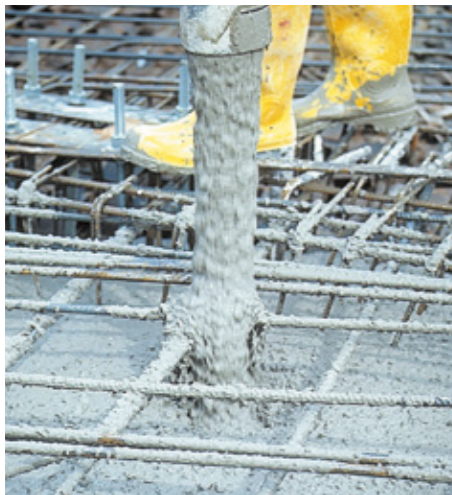
Casting a concrete floor slab
