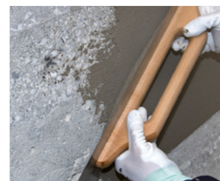
Application of thixotropic smoothing and levelling compound on a wall
