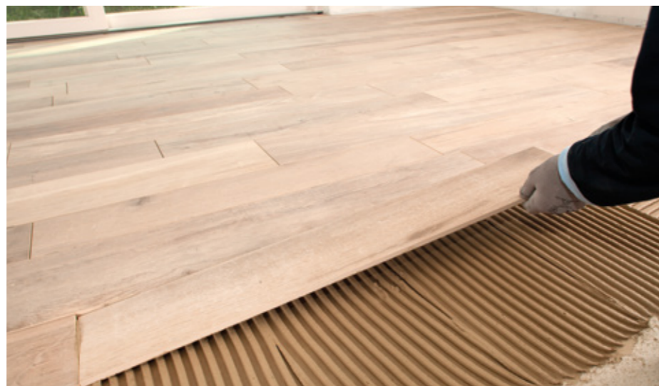
Installing large format tiles with a wood-effect finish
