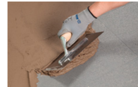
Application of thixotropic smoothing and levelling compound on a floor
