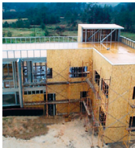
Structure made from OSB panels
