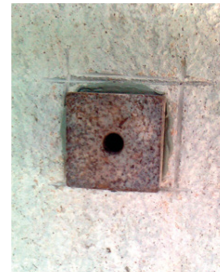
Bonding a test sample to carry out a pull-off test on render
