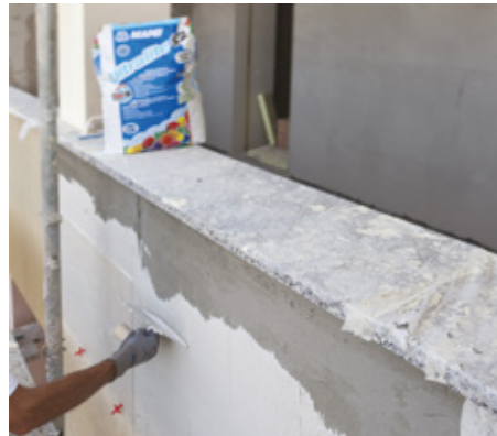
Spreading adhesive on the substrate
