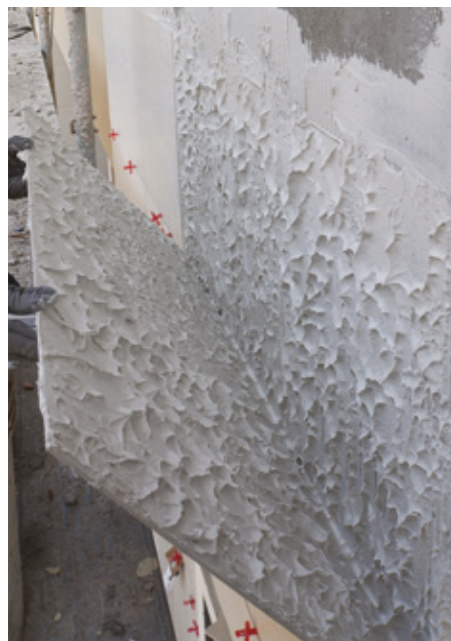
Checking complete wetting of the back of the tile
