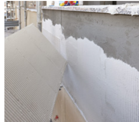
Installing a tile
