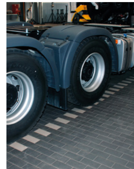
Flooring subjected to dynamic loads
