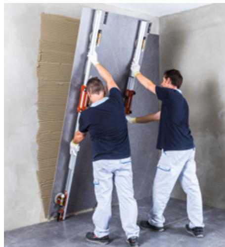
Handling and manoeuvring thin tiles
