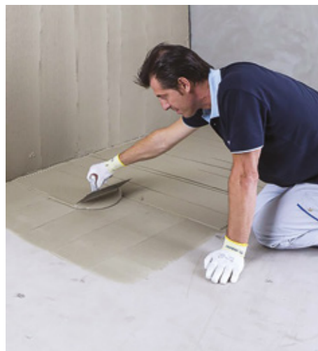
Double-buttering application of adhesive for a thin tile
