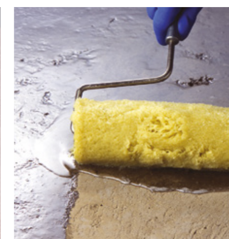
Application of adhesion promoter on an absorbent substrate
