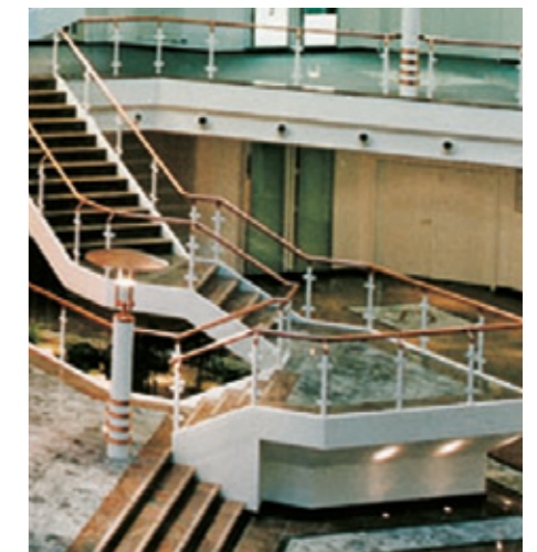
Installing ceramic on metal substrates
