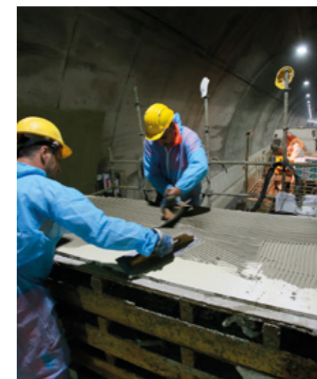
Spreading adhesive on the back of the tiles
