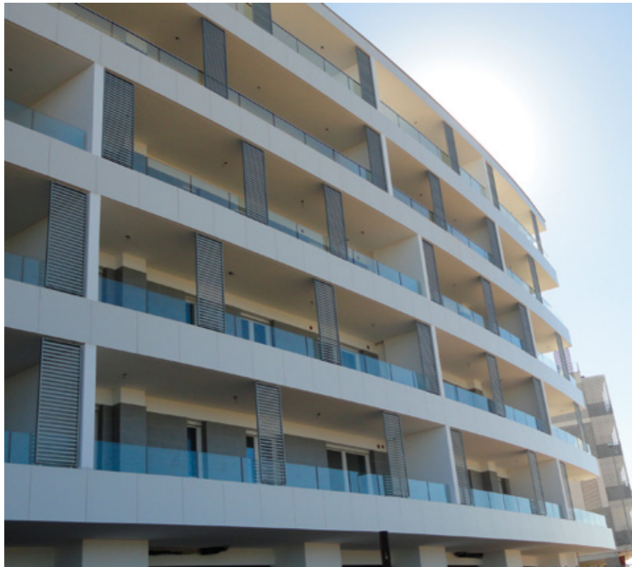
Installing thin tiles on a façade; Sant'Anna apartment complex, Bari
