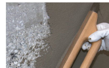
Application of thixotropic smoothing and levelling compound on a wall
