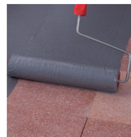
Application of ECO PRIM GRIP on a non-absorbent substrate
