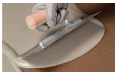
Application of MAPELASTIC TURBO
