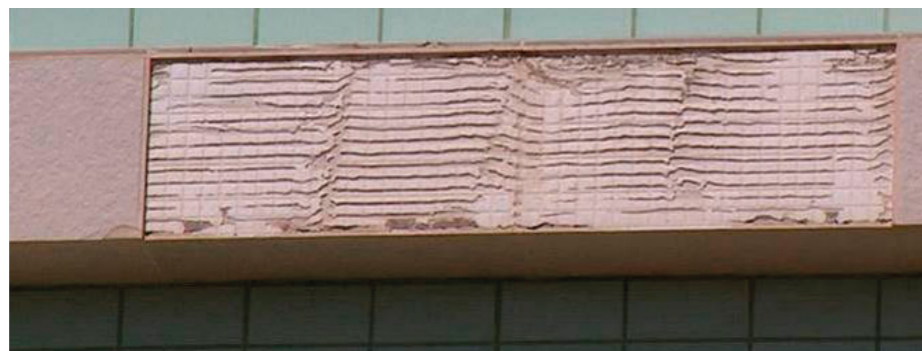
Installation during windy weather. The skin formed on the surface of the adhesive inhibits it from being transferred on the back of the tile.
