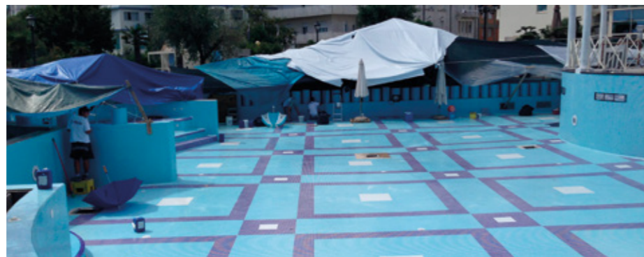
Installation carried out on surfaces exposed to the sun: surfaces must be protected from direct sunlight when the surrounding temperature is high
