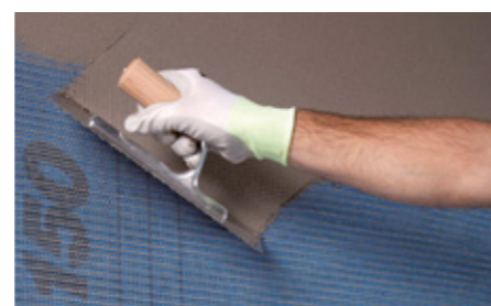
Application of MAPELASTIC
