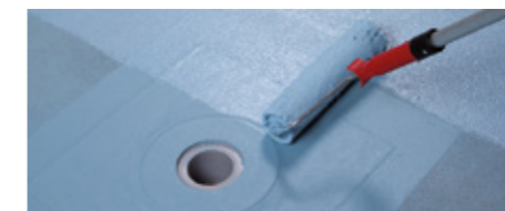
Spreading MAPELASTIC AQUADEFENSE with a roller
