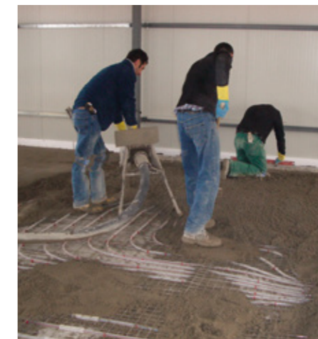
Sub-layer with the heating elements for the system embedded in TOPCEM PRONTO
