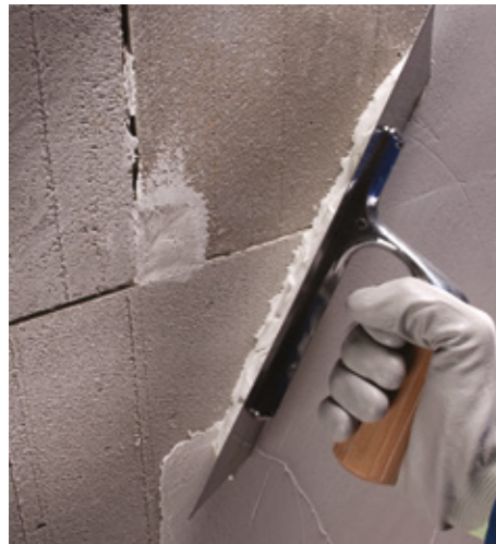
Application of skimming compound on lightweight concrete blocks
