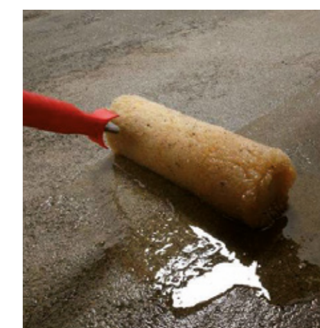
Application of consolidating-waterproofing primer
