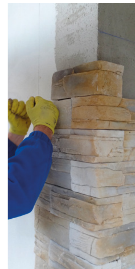
Installing stone veneer with an “exposed” finish
