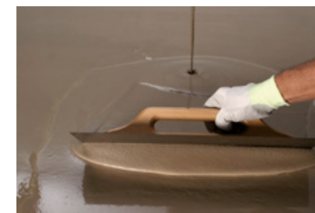
Application of self-levelling smoothing and levelling compound
