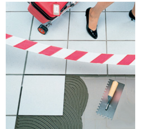
Rapid installation of ceramic flooring in a shopping centre
