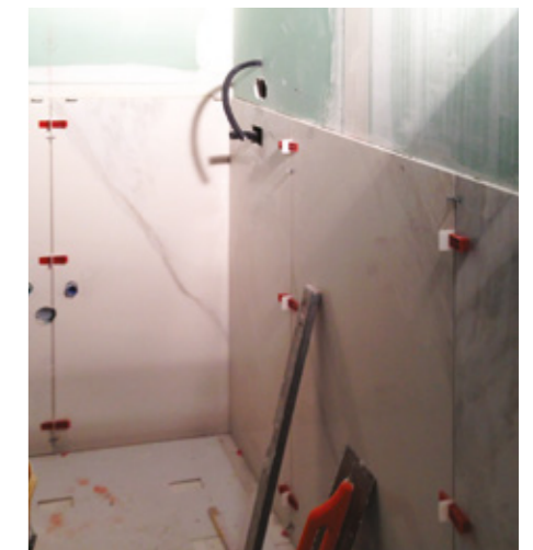
Installing ceramic on plasterboard panels
