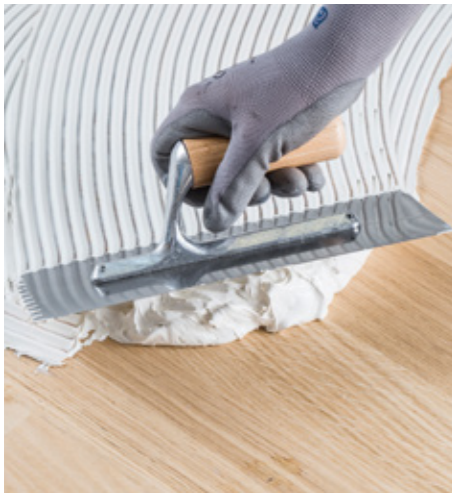
Installing ceramic on a wooden floor
