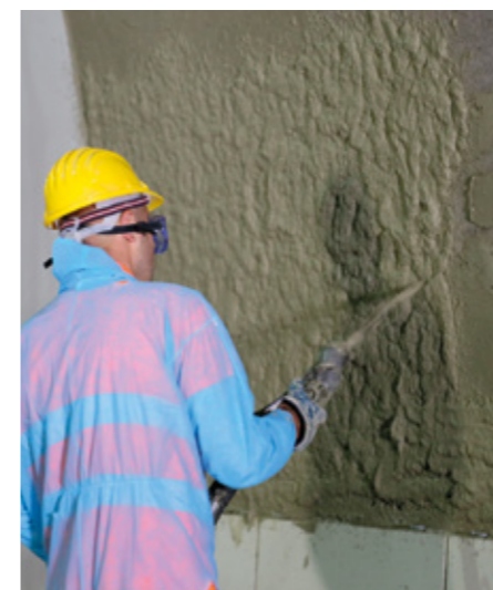
Spray-application of adhesive on the installation bed
