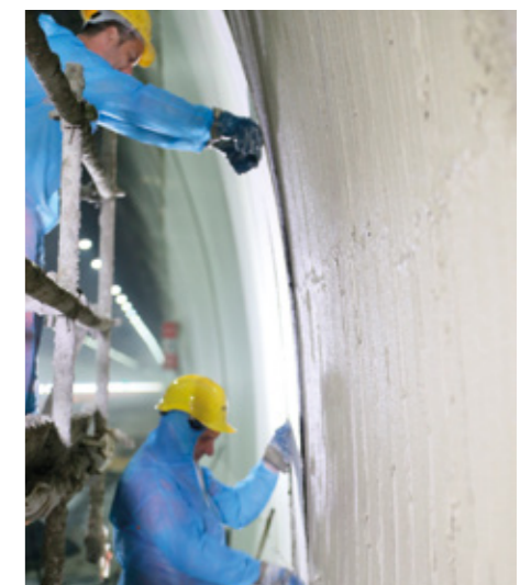
Bonding a tile to a tunnel pier
