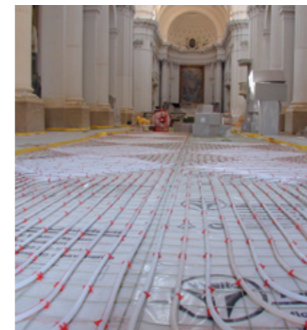
Installation of pipework in an underfloor heating system
