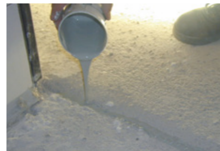
Sealing cracks in a substrate with EPORIP
