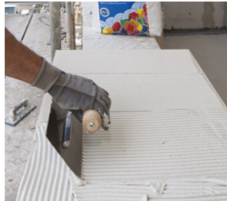
Spreading adhesive on the back of a tile
