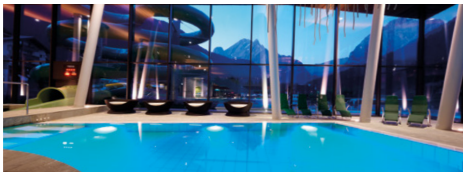
Dalaondes, Canazei. Installing ceramic in a swimming pool
