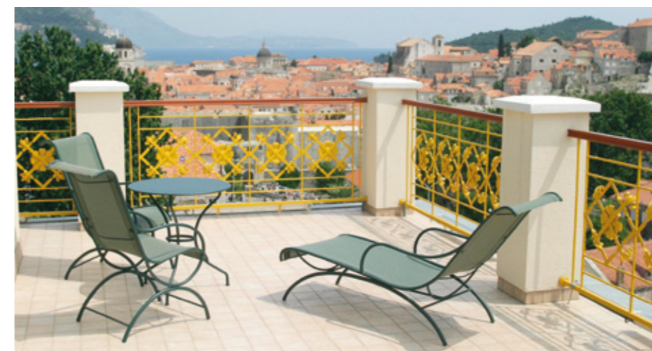
Hilton Imperial, Dubrovnik. Installation of ceramic on terraces and balconies
