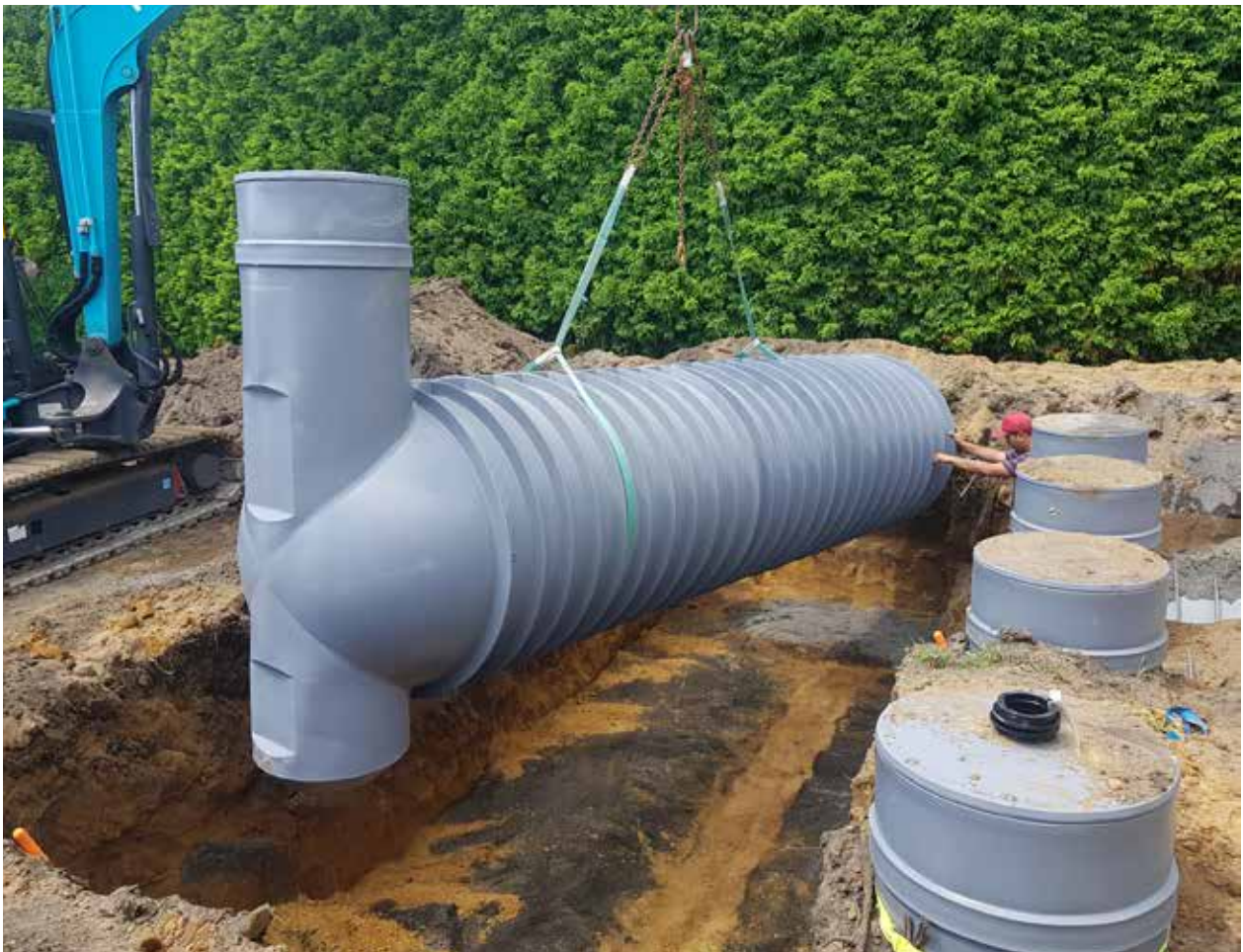
7,000L tank install part of total - 47,000L drinking water system
