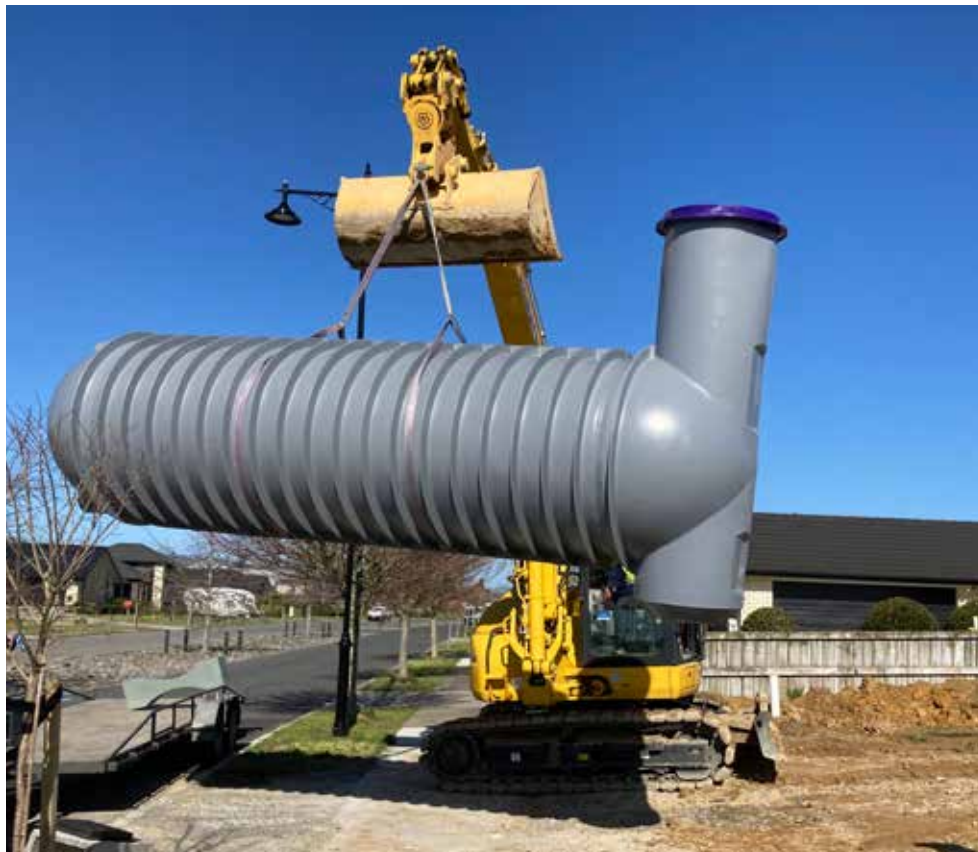
5,000L Under drive install
