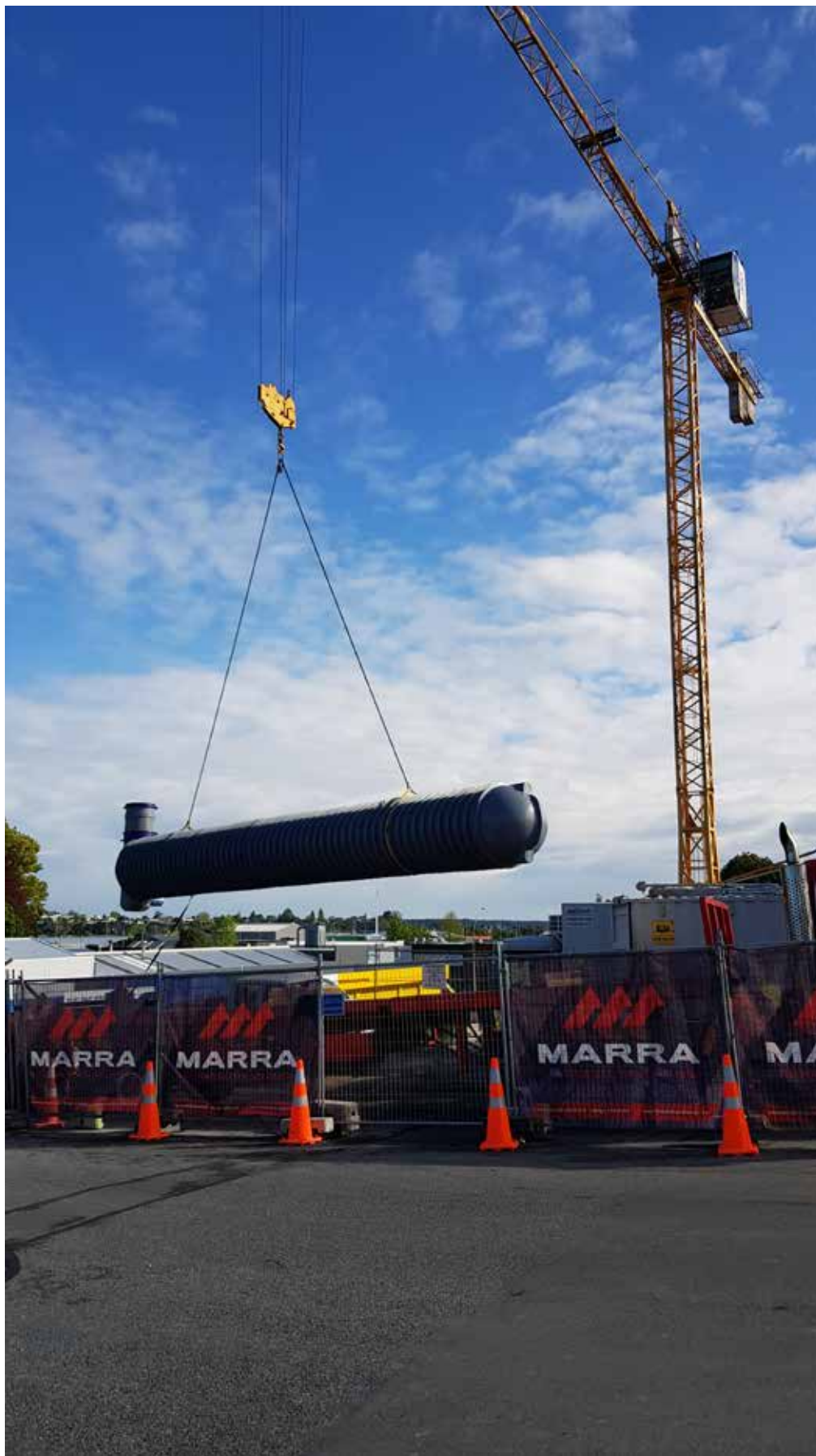
12,500L Under drive install
