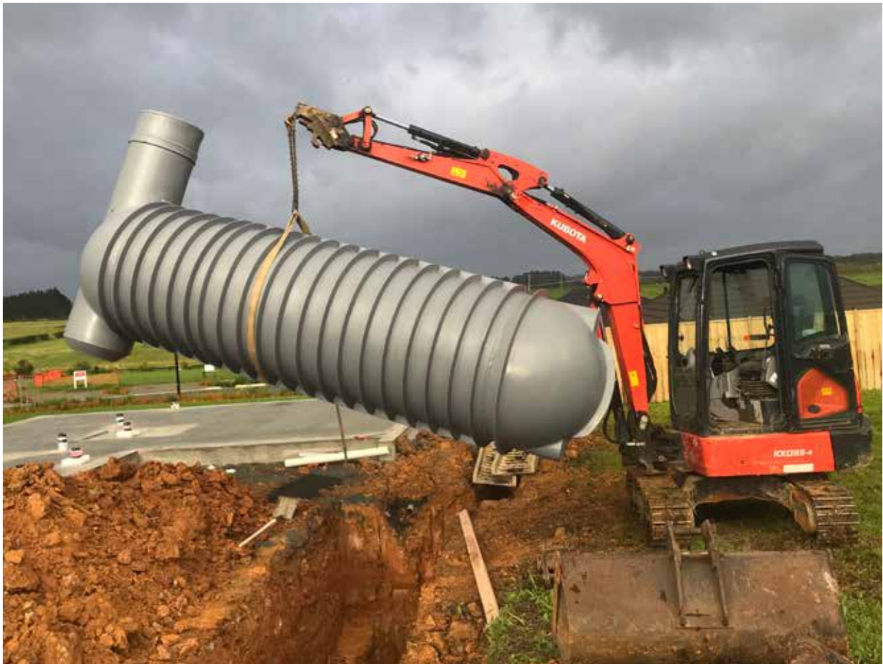
6,000L under garden install
