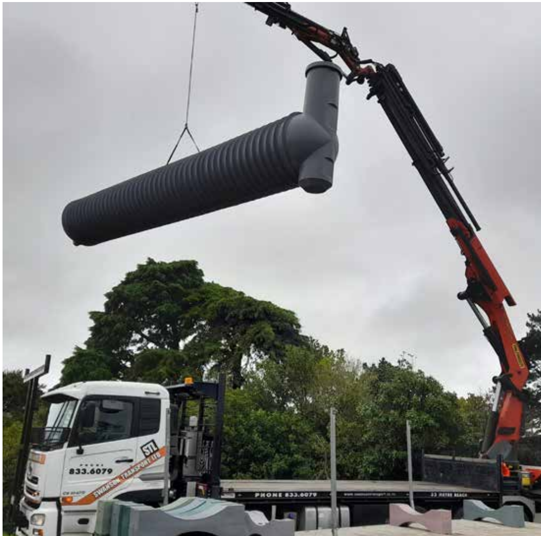
10,000L Under drive install
