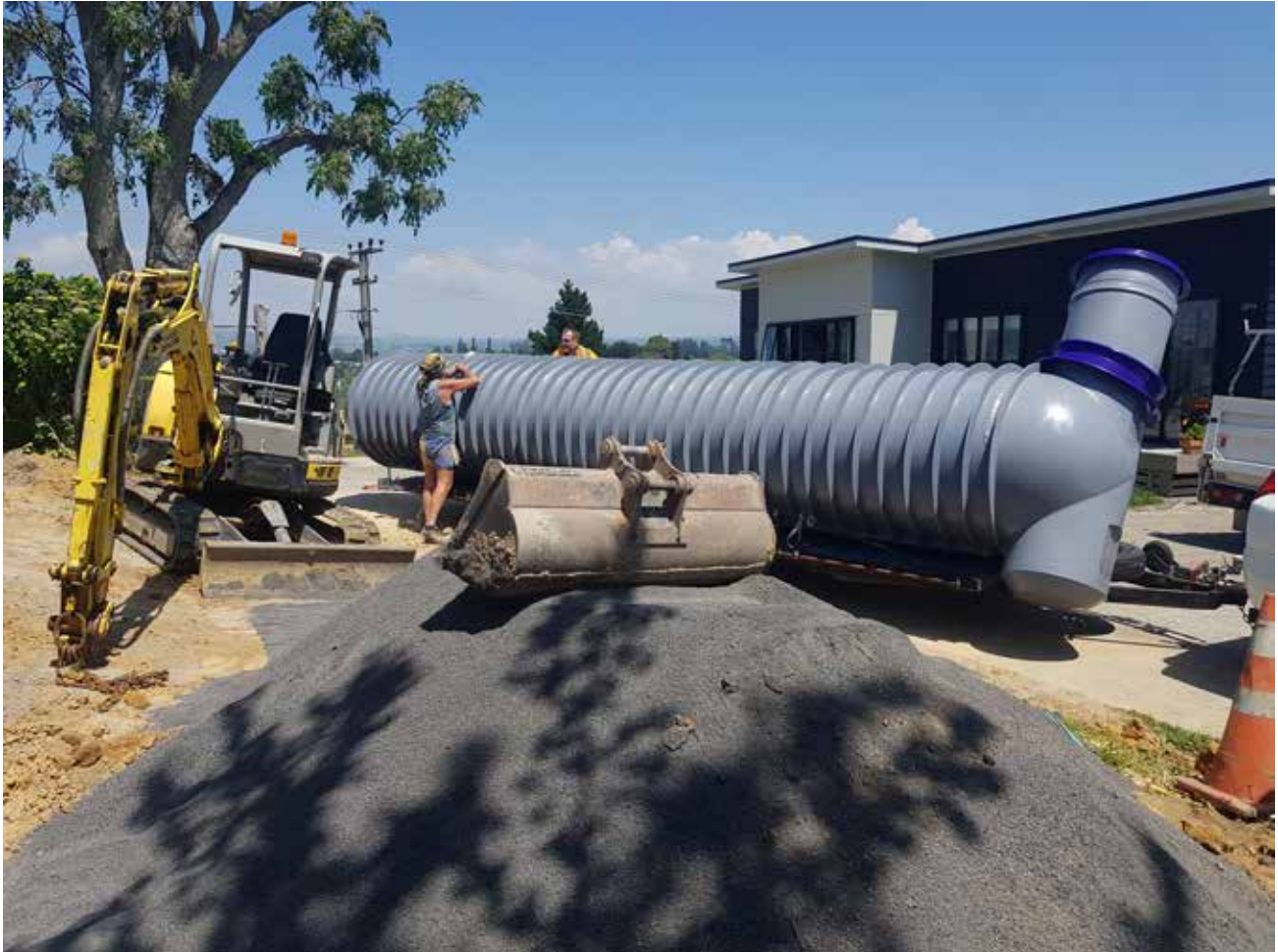
8,000L Drive install
