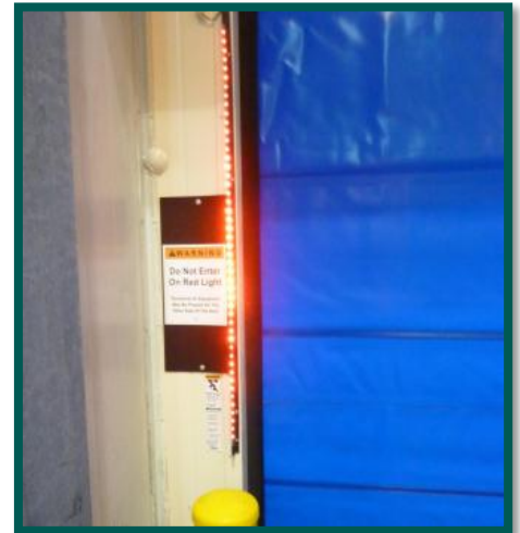
WARNING LIGHTS ALERTS PERSONNEL TO APPROACHING TRAFFIC WHERE THERE IS OBSTRUCTED VISIBILITY
