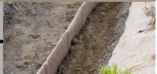
Backfill over the 200mm flap
