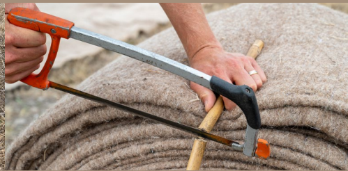
Cut a pilot guide pole to 250mm
