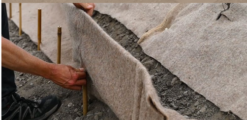
Slide pockets over poles leaving the 200mm flap uphill
