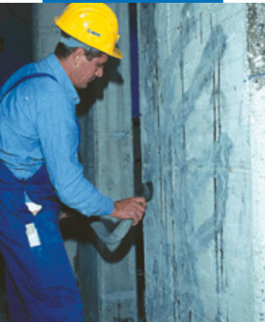
Preparing the substrate
