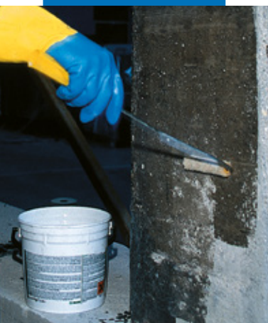
Applying a second coat of MapeWrap Primer 1
