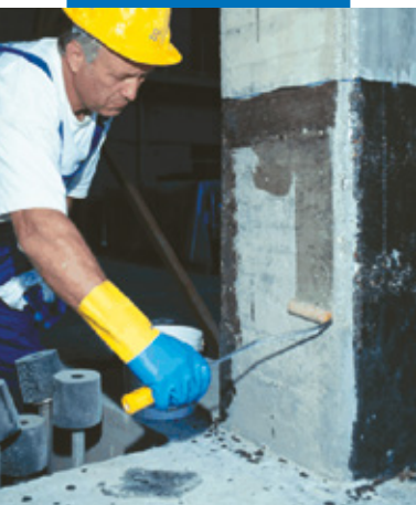
Applying a first coat of MapeWrap Primer 1
