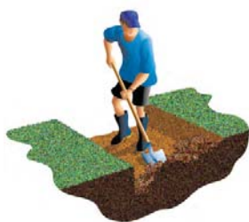
EXCAVATE & PREPARE THE SUB-GRADE
