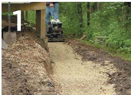
1 PREPARE THE BASE LEVELLING PAD
