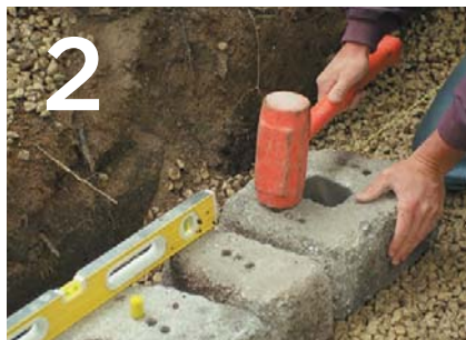
2 INSTALL THE FIRST COURSE & PINS
