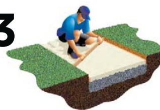
PREPARE THE SAND BASE
