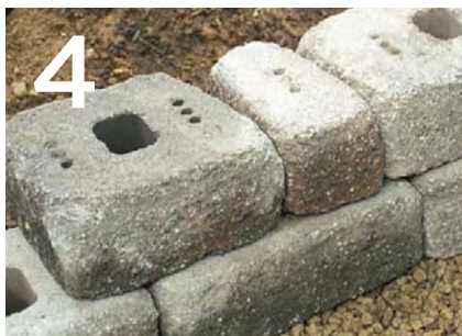
4 INSTALL ADDITIONAL COURSES (NO MORTAR REQUIRED)
