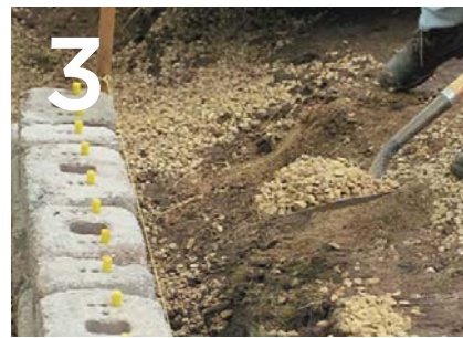
3 BACKFILL & COMPACT
