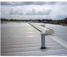
The Colt solution was to ventilate the factory by utilising the powerful natural currents already present within the building. This was achieved by placing electrically controlled Multi-Function ventilators along the ridgeline to allow the hot air to escape, and placing SeeFire operable louvred ventilators at low level to allow cool fresh air to enter as replacement.
