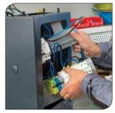
Insert wired protection kit in the floor base.
