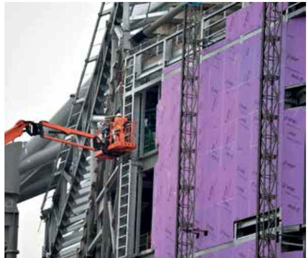
Gypsum sheathing has been widely used for many years in harsh overseas climates.
