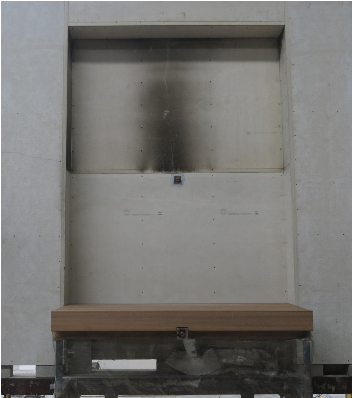
Figure A6.1: Exposed face of specimen before commencement of the fire-resistance test
