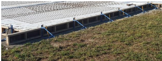
Fig 6 Example Boxing with shutters
