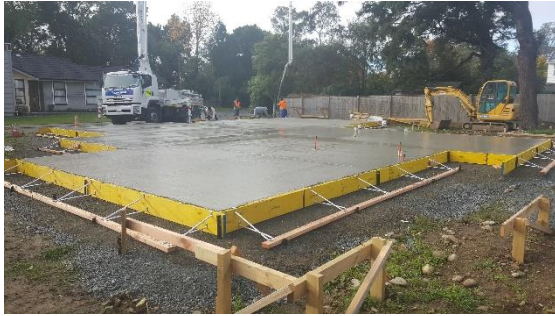
Fig 5 Example Boxing Setup
