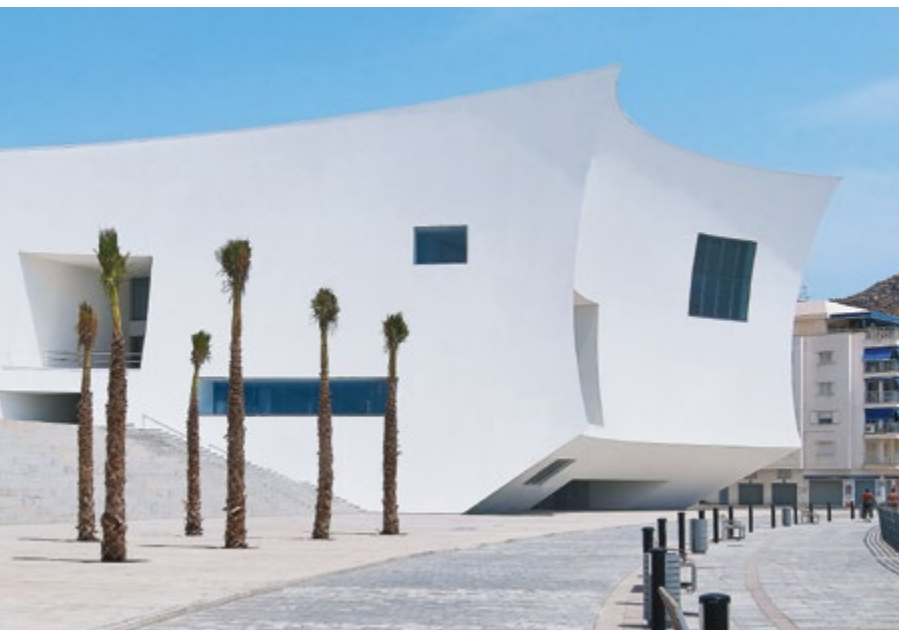
Auditorium and congresses, "Infanta Doña Elena", Aguilas /Spain Architectural firm: Barozzi Veiga, Barcelona
