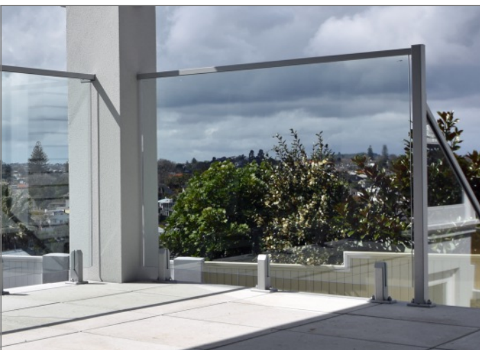
Juralco Edgetec® Mini Post, Top Fixed. Showing the Interlinking Top Rail and the use of a Top Mounted Edge Post and Brackets back to the structure
