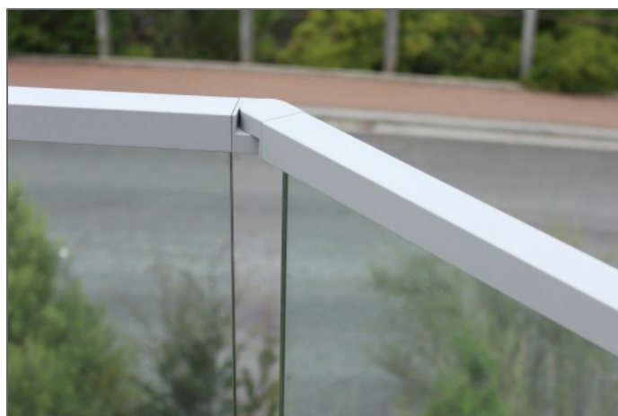
Interlinking Top Rail. Angled Joint
