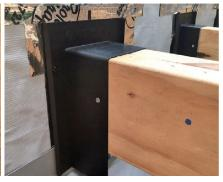
Tape sides and top of Pro-Joist back to underlay. Pro-Joist Pro-Joist to be painted or protected from UV by scriber. overhangs joist by minimum of 35mm.
