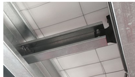
SE105HP-2PBP plates attach to the SE015HP mounting plate
