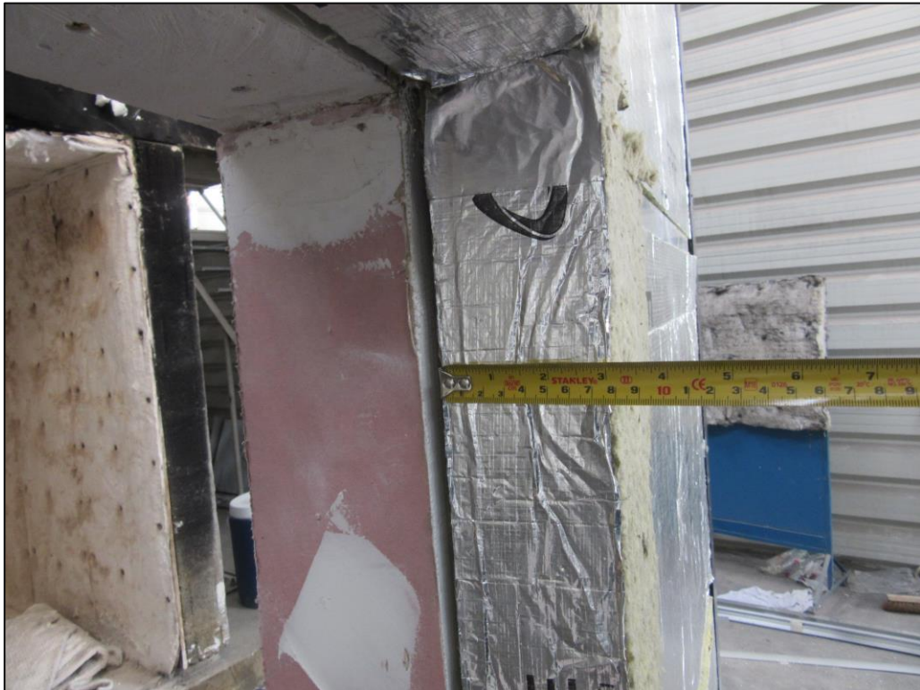
Picture 3: Cavity fire barrier along the window aperture.
