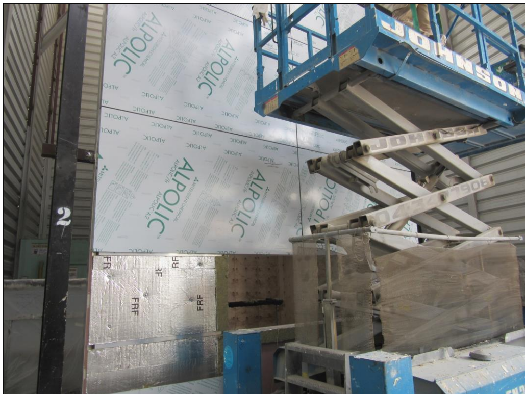
Picture 8: Alpollic FR ACP's fixed onto the framing system.
