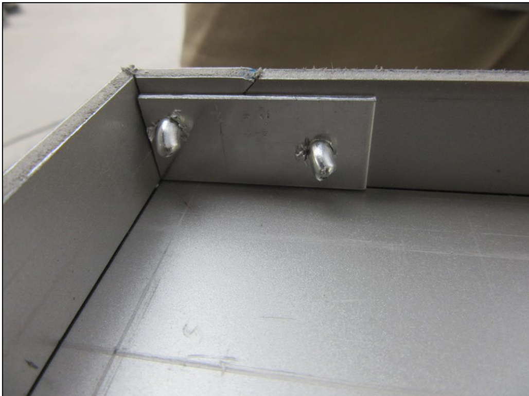
Picture 6: Aluminium strip at 45° corner joint of ACP's.
