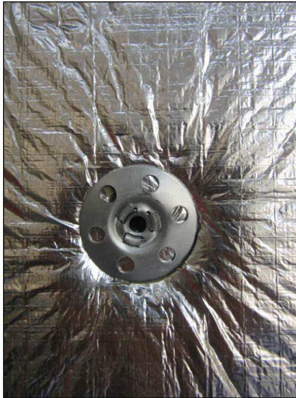
Picture 5: External insulation slab fixing anchor.
