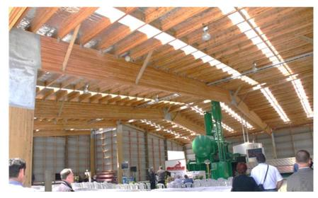
cut and fixed to the Glulam columns in our factory. A typical frame arriving on site consists of two Glulam columns with gussets attached and one continuous pitched rafter member. The rafter is able to extend beyond the columns thus providing an overhang. For large spans the rafter can be supplied in two sections with an apex gusset. All members are pre-finished in factory and require no further attention once erected in industrial buildings.
