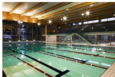
Diocesan School (Auckland). Post Tensioned box beams 27m span over indoor swimming pool.
