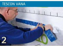
Seal the membranes at overlaps without strain or loading, using TESCON VANA adhesive tape. The tape should be applied centrally and pressed down firmly using, for example, pro clima PRESSFIX.
