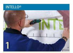
The INTELLO® airtightness membrane is laid on the interior, over the insulation. Bonding with adhesive tapes should be on the smooth printed side. Staples should be 10 mm wide and 8 mm long and set at a maximum distance of 100 mm-150 mm.
