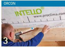
The liquid adhesive ORCON is applied to join the INTELLO® membrane to concrete or wooden frames. Do not press the adhesive completely flat.
