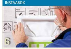
The airtightness box for power points and light switches is cut and fitted into the INTELLO® layer and then sealed by using TESCON VANA to create a seamless airtightness system.
