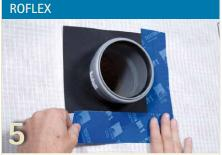
ROFLEX pipe grommets are affixed using TESCON VANA. Press firmly to secure the adhesive tape.
