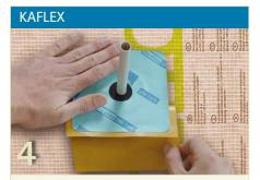
If pipes or cables penetrate the airtightness layer, they too must be securely sealed.
