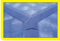
Starting at the bottom of the hip, position the first trim hanging over the edge of the shingle and
