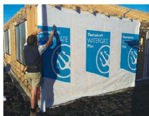
Fix Watergate Plus securely to the frame.
