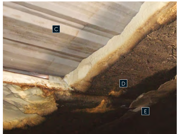
C: Temporary roof covering over hole in roof.
