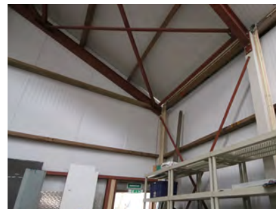
No heat transfer damage to interior of adjacent property (building A).
