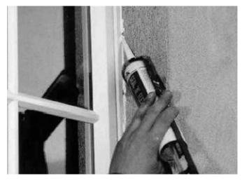
B: apply a flexible seal to the gap between the top and sides of window frame and masonry wall. Do not seal along the bottom of the window frame.
