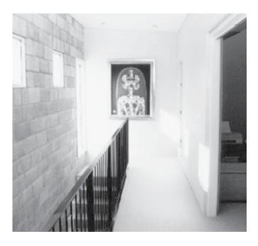
Paint over bare blockwork is a relatively low cost solution. This provides a uniform colour to the wall and still allows the mortar joints to be seen. It is important that the walls are as dry as possible before applying the paint. If any excess moisture is trapped, it is likely to bubble the paint over time. In order to hide the block lines, a high-build elastomeric coating with a levelling coat can be used.
