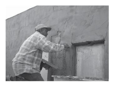
it makes a slight hollow sound. After this preparation coat, it is common for two or three coats of plaster to be trowelled on. It is even possible to spray the plaster on which speeds up the process. The top coat of the plaster can be coloured to match the paint just like an undercoat.
