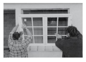
Ensure that the window frame is located accurately and square in the opening. This will ensure a uniform gap around the frame for further application of sealant.
