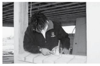
Apply a waterproofing membrane around head, jambs, and sill. This waterproofing membrane should cover the entire thickness of the wall and be extended a minimum of 50mm on the exterior face around the penetration.
