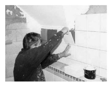
• It is of utmost importance to ensure that blockwork is dry before application of tiles as any shrinkage movement will reflect cracks in the surface due to their brittle nature.
