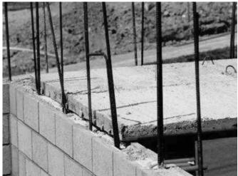
The props may be removed once the concrete topping has reached a compressive strength of 15MPa. This is
