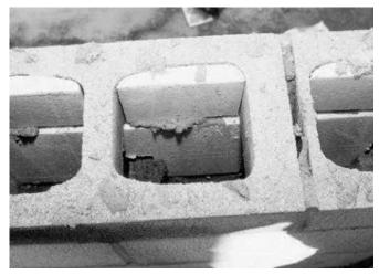
the vertical steel. This will allow the blockfill to finish flush with the outside face of the blocks. It is important to ensure that the formwork is braced adequately to prevent blow out under grout pressure. Often small gaps are left in the formwork at the washouts to allow the blockfill to flow out. These are to confirm that the blockfill has fully filled the wall and are plugged once confirmation has been made.
