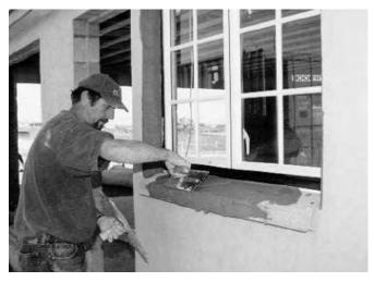
With the paint system, it is very important that the paint coat is applied over the flexible sealant up to the joinery. This provides one extra defence against moisture ingress. The Architect or Designer should fully detail the weatherproofing procedures for window openings.
