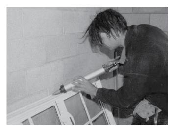
Fit joinery leaving a 5mm gap between the window frame and masonry rebate.
