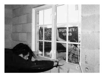
A: Once the window is fixed and square install backing rod and foam airseal to the interior of the jonery.
