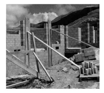
Typically bracing at 3m centres is recommended in line on both sides of the wall.
