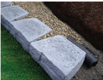
5. Lay drain coil and drainage aggregate
