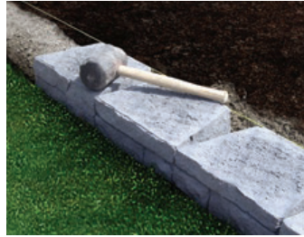
4. Lay first layer
