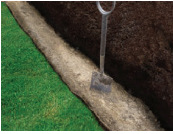
1. Mark out and dig trench
