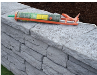
9. Place capping stones on and glue down if you wish
